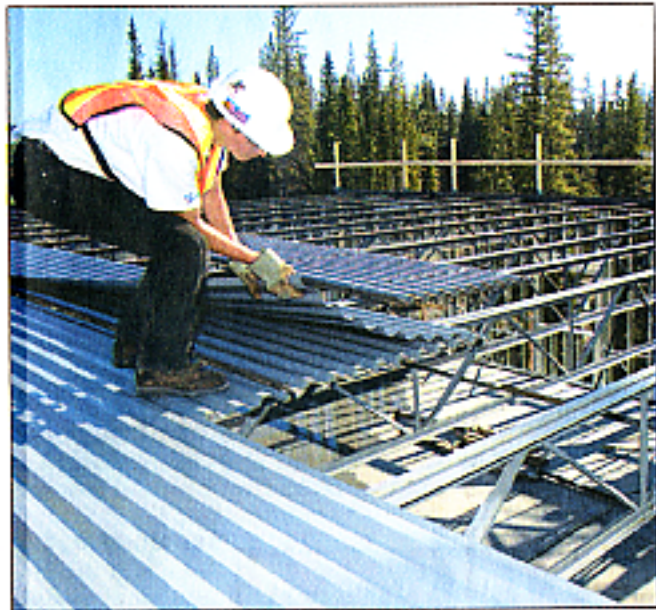
Photos: Mikael Kjellstrom, Calgary Herald Above, a worker lays down metal decking at The WedgeWoods of New Discovery, Chateau I. Left, construction manager Frank Castronuovo at the site.
